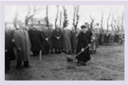
The turning of the sod on the new vocational school in Carndonagh by Fr Bonner, P.P. circa 1957/58.
